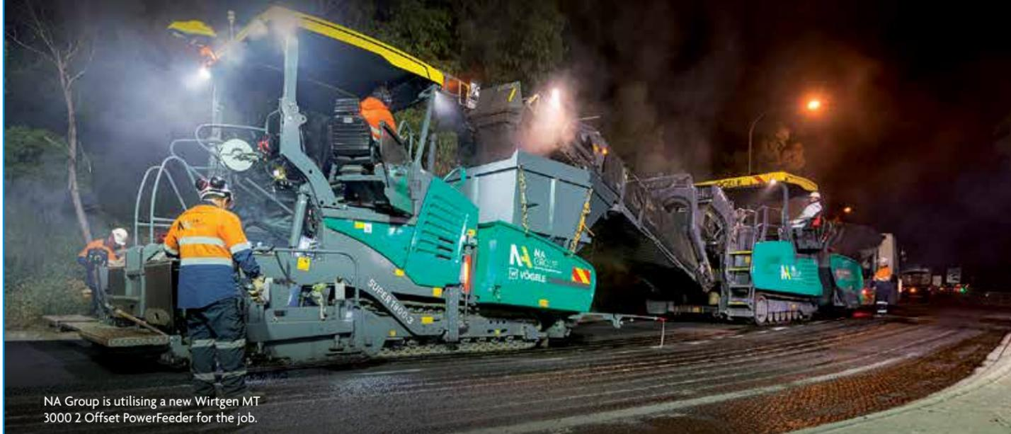
NA Group is utilising a new Wirtgen MT 3000 2 Offset PowerFeeder for the job.
